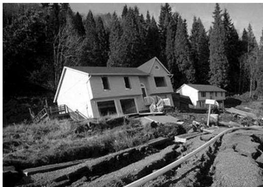
*Figure 7 : House destroyed by reactivated landslide in 1998 in Kelso, Washington*
