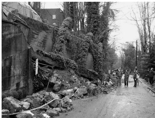
*Figure 8 : Plugged up drainage system of 100 year old house causes wall to collapse and crush two cars in Portland, Oregon, in 2006*
