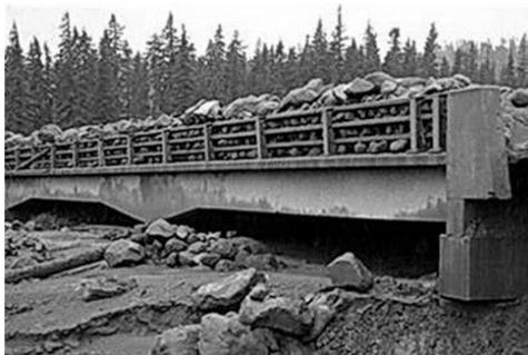
*Figure 3 : White river bridge on highway 35 buried by debris flow of 2006, Mt. Hood, Oregon. Photo courtesy of USFS*
