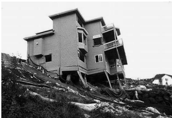
*Figure 5 : House on toe of ancient landslide reactivates as a slump during Portland storm of 1996*
