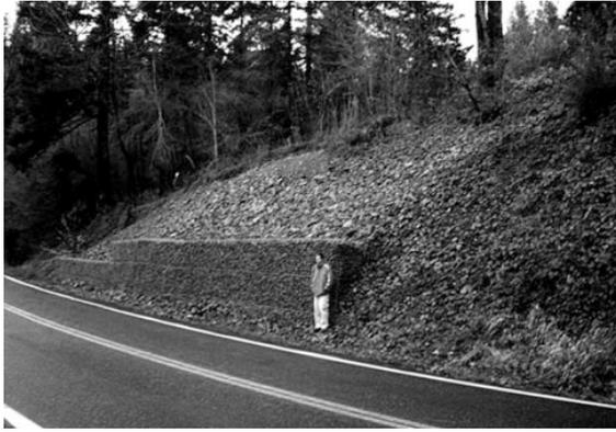
*Figure 2 : Gabion wall—normal mitigation for earth flows in Portland's West Hills*
