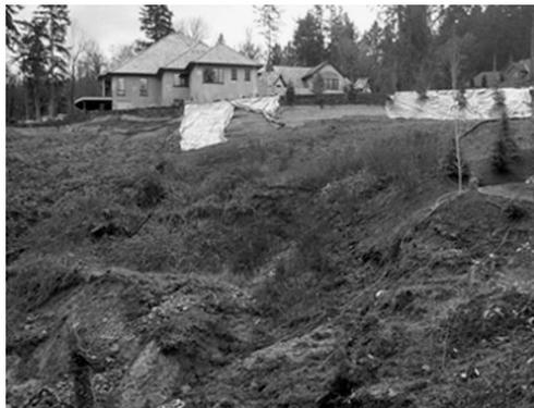
*Figure 14 : Romeo and Juliet House is destroyed by an ancient landslide that reactivated in 2006*
