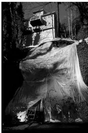
*Figure 1 : Landslide in Portland West Hills—cause a leaking pipe*
