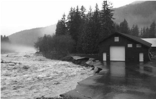
*Figure 10 : Nisqually River eroded into the Longmire service center for the Mt. Rainier National Park, 2006 debris flow. Photo courtesy of USFS*
