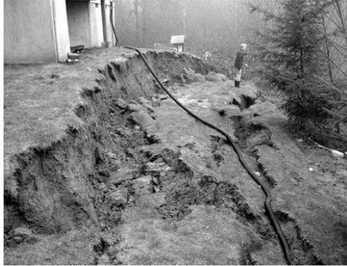
*Figure 13 : Toe of reactivated landslide slump at Newell Creek Apartments in Oregon City, Oregon*
