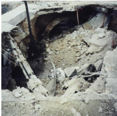
Figure 7: Metro of Athens. A major collapse at the zone of weak "athenian schist". The face had a zero stand up time in front of the cutter head of the TBM and a raveling occurred through its openings inside the machine
